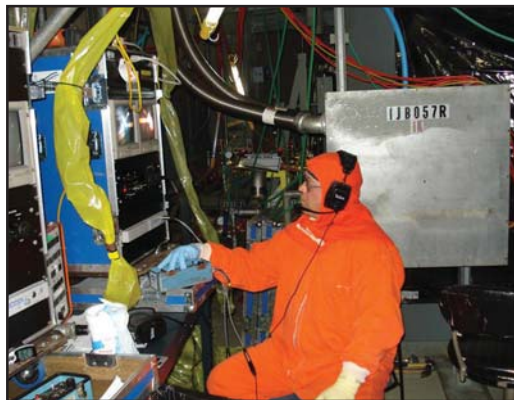
PCI Welder Bob Hopper Welding on Braidwood Unit 1 Surge Line Nozzle SWO
