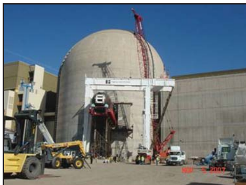
Replacement SG on Outside Runway being Transported into Containment
