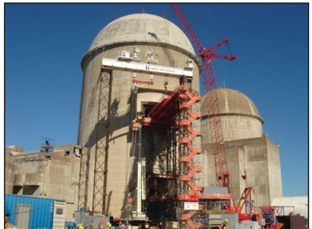
Comanche Peak Steam Electric Station Unit 1
